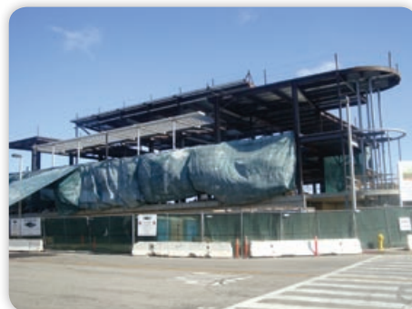
Roof and Outdoor Viewing Terrace Completed
