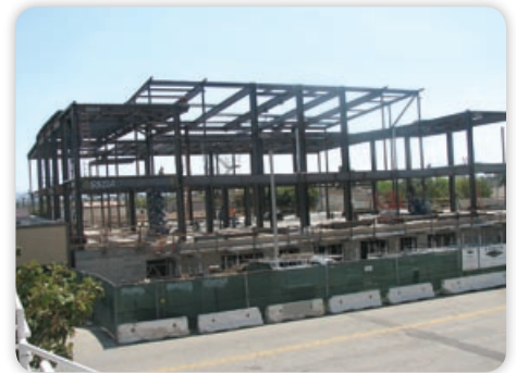
Community Center Building Skeleton
