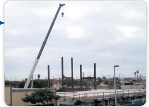
Placing Second Floor Steel Columns
