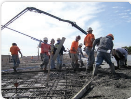
Workers Spreading First Deck Cement
