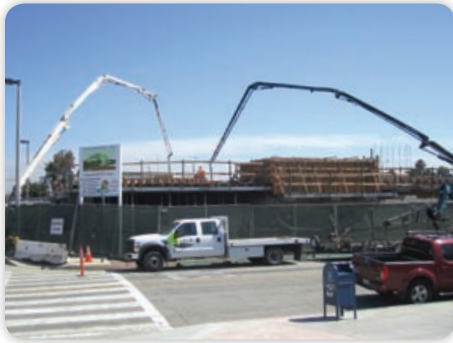
Twin Pumps Filling the First Deck
