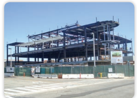
Center Waiting for a Roof
