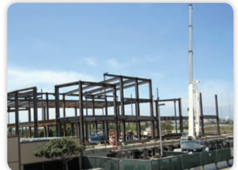
Third Floor and Roof Construction Underway
