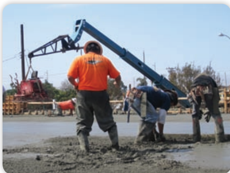
Workers Smooth and Level First Deck
