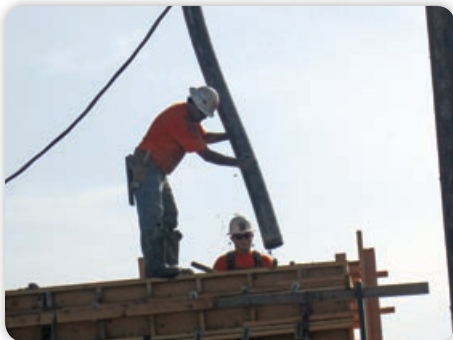
Workers Directing Cement Flow
